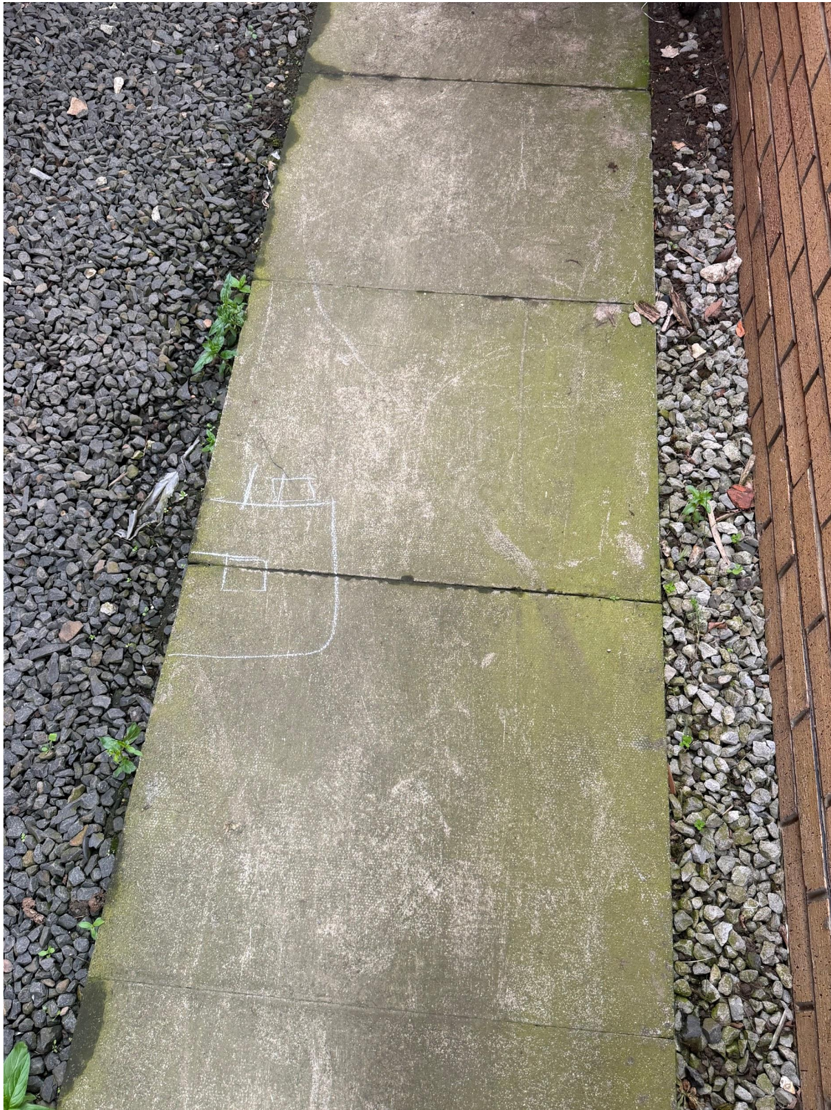
Proposed railing post location marked in chalk
