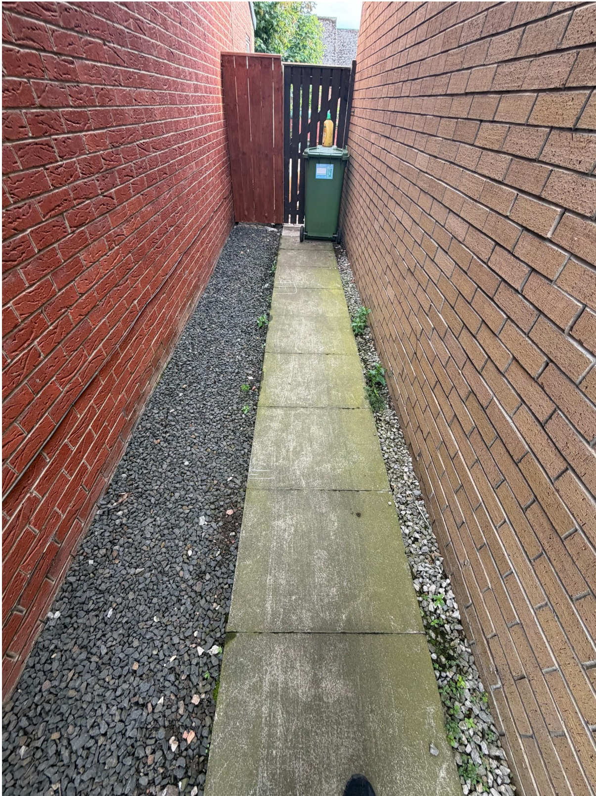
Proposed railing post location marked in chalk
