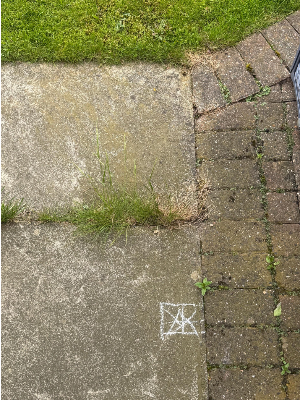
Proposed railing post location marked in chalk
