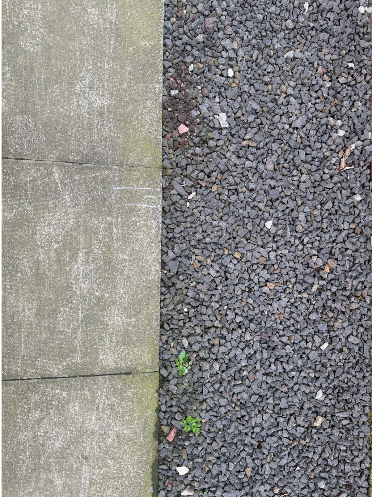
Proposed railing post location marked in chalk
